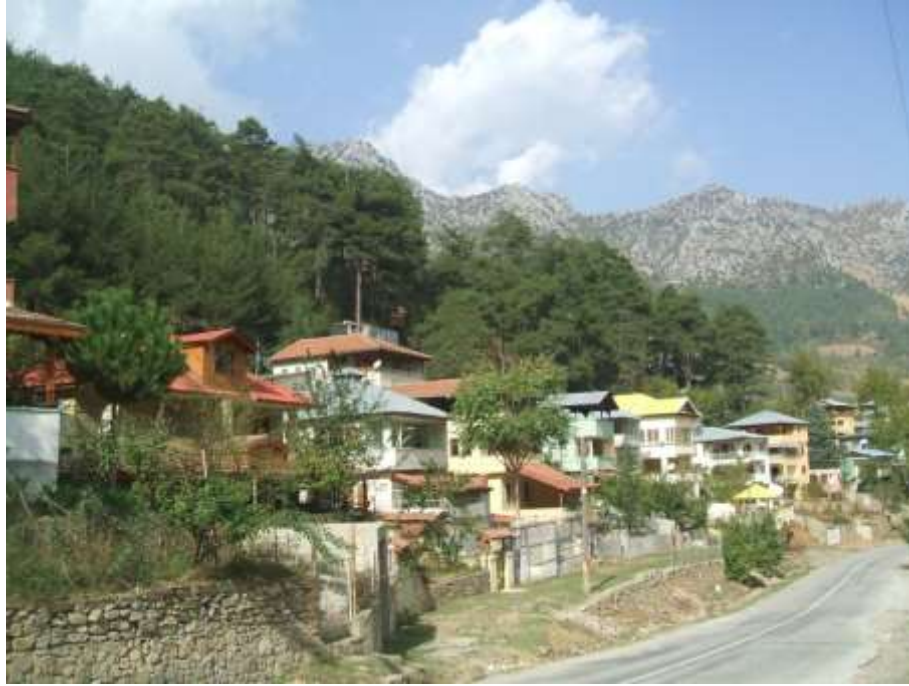
Figure 4: Reinforced Concrete Summer Houses in Horzum Yayla
